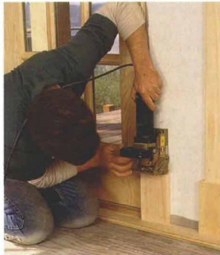
Slotting in place. To deal safely with a small piece, this carpenter installed the plinth block first and slotted it in place (above). In the photos below, he adds a biscuit, then the casing.
