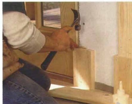
Slotting in place. To deal safely with a small piece, this carpenter installed the plinth block first and slotted it in place (above). In the photos below, he adds a biscuit, then the casing.
